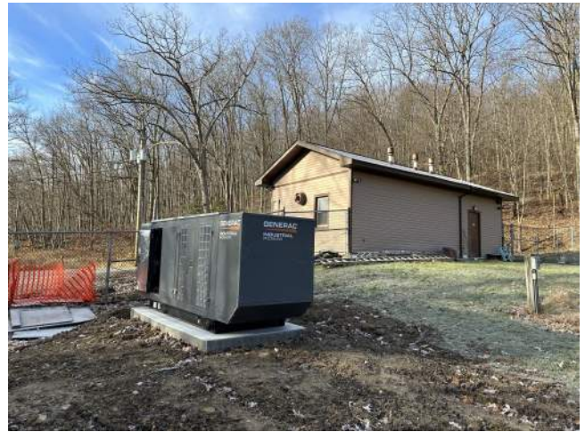
Black Moshannon State Park — Installation of 140kW Propane Generator System
